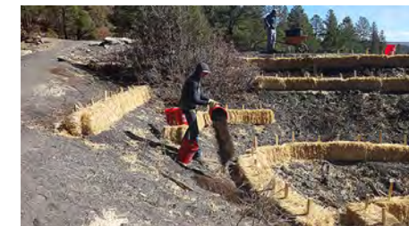
Contractor adding compost and wood chips before straw bale terraces.
