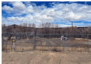
Ramel Family Farms greenhouse grading
